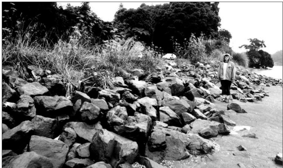
of these poses particular problems. Sea walls reflect waves and cause greater turbulence and erosion immediately in front of them; they often fail through being undermined by such erosion; and they often fail to retain the beach material behind them and the erosion continues despite their presence. Specialist engineering advice is needed for any of these structures.
