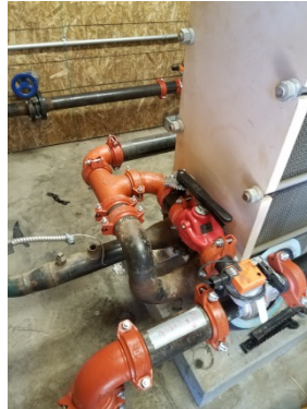
Figure 12: New Heat Exchanger for Middle and Elementary Schools
