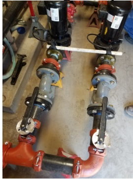
Figure 13: Elementary School Circulating Pumps in New Heat Exchanger Building
