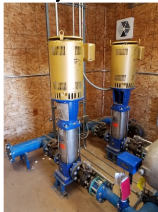
Figure 16: Injection Well Pumps
