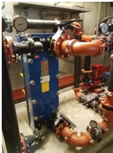
Figure 15: High School Heat Exchanger
