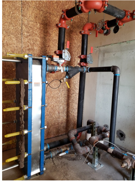
Figure 6: Wood Shop Heat Exchanger
