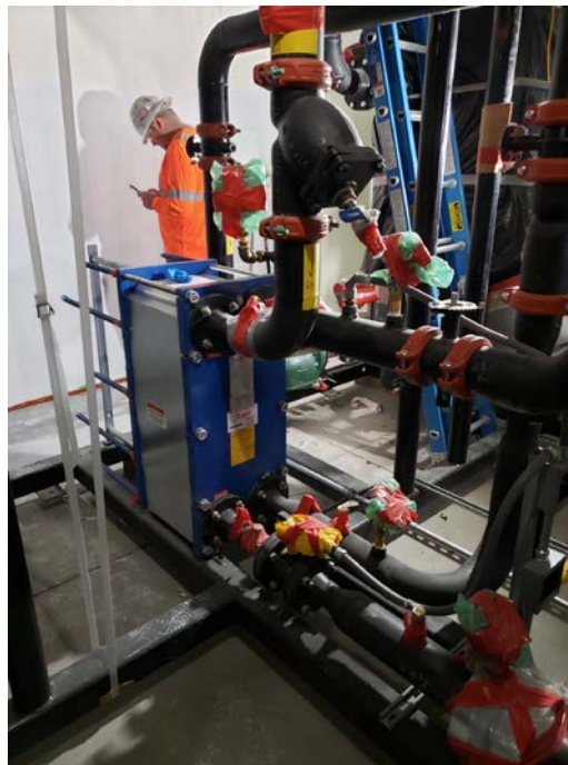
Figure 4: Modoc Medical Center Heat Exchanger
