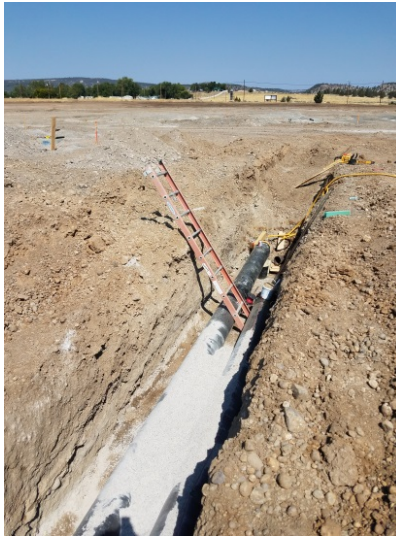
Figure 2: Geothermal Piping Installation
