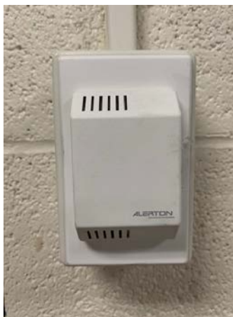
Figure 12: Typical Thermostat Control Unit
