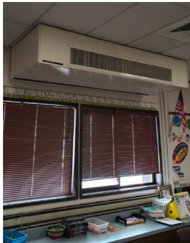
Figure 11: Typical Classroom Heating Unit
